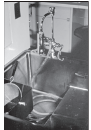
FIGURE 17. Atmospheric vacuum breaker in plumbing supply system.
