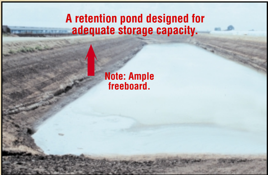
Do construct retention ponds with sufficient storage capacity. Accommodate facility washwater, manure and bedding, normal rain including runoff, and the 25-year, 24-hour storm event. Provide flexibility for management to apply liquid manure at appropriate rates. Be sure pond sidewalls and bottom are at least 10 percent clay and not more than 10 percent gravel.
