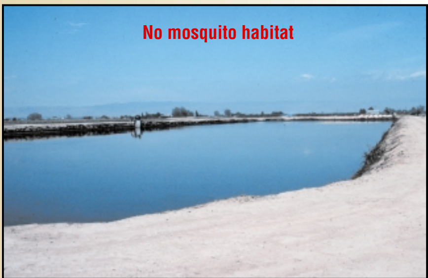
Do prevent mosquito habitat. The level of the pond can be raised and lowered to eliminate breeding areas.
