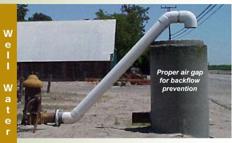
DO have adequately designed backflow prevention from well heads.
