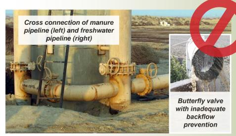
DON'T cross connect manure and freshwater pipelines without adequately designed backflow prevention. Do not use faulty, inadequately-sized, or adapted valves in manure systems.
