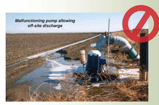
DON'T allow poorly maintained equipment to result in off-site discharge of manure water.
