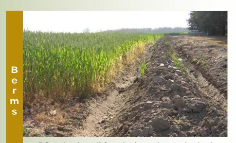
DO maintain well-functioning, adequately sized berms free of erosion and rodent damage.
